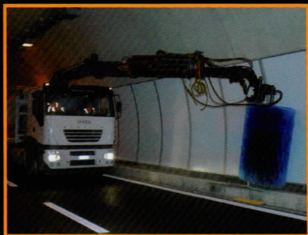
Rotolavaggio of ceramic painted aluminum panels.
