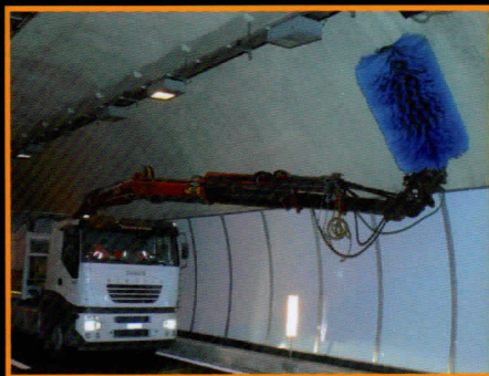
Rotolavaggio of ceramic painted tunnels sides and ceilings.
